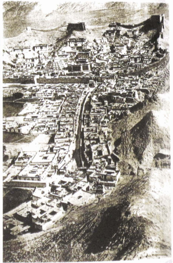
Pl. 11 From atop Gyantse Dzong's citadel a sweeping view of the town where Gergan Tharchin would live and teach for more than two years, 1921-3. The main thoroughfare is divided by a long "mendong," and the large Palkhor Chhode Monastery sits enclosed within its walls that fills up the upper end of the photo. Note also the location of the renowned golden-roofed Chorten in the upper left section of the monastery wall (see next Plate).
